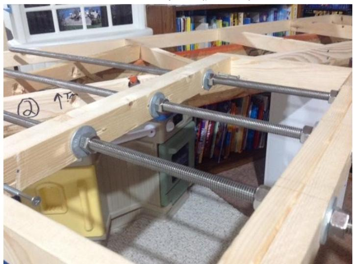
Photo 2 shows the carriage bolts extending from the left into the peninsula which allows it to be free floating and wheelchair accessible.
